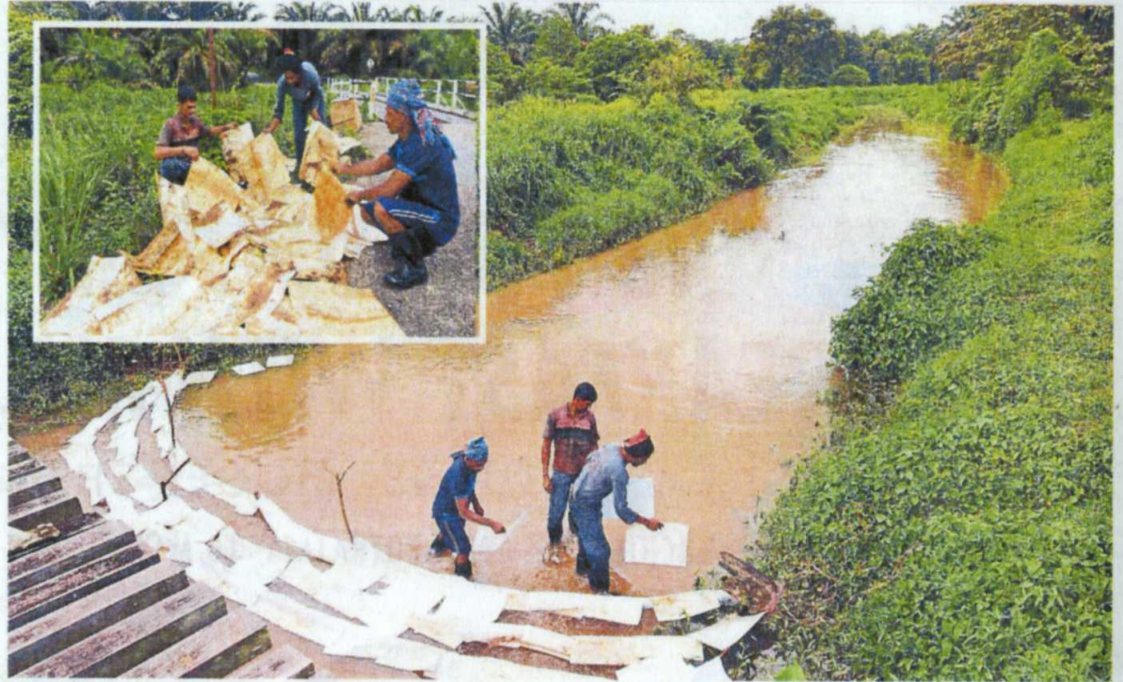
Fighting pollution: Workers from the factory believed to be the cause of the oil spill arranging fabric sheets to contain oil in Sungai Johor and (inset) collecting spent sheets.
